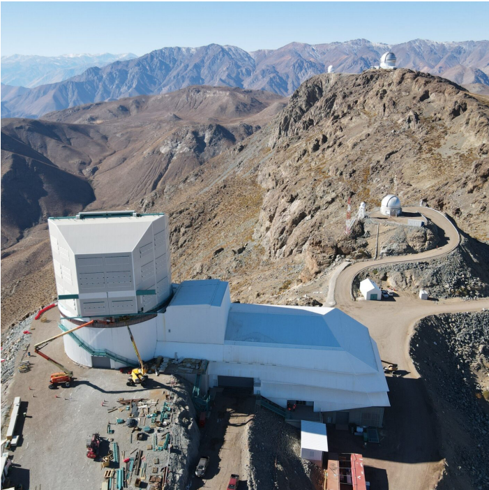
Rubin Observatory, which will take nearly a decade to complete, has a unique appearance compared to other observatories due to its large support building that will act as a maintenance shop for the supersized camera and telescope.
